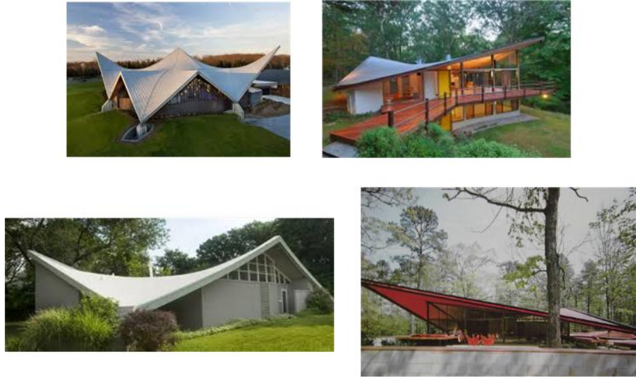
Figure 4. Roof structures based on hyperbolic paraboloids
