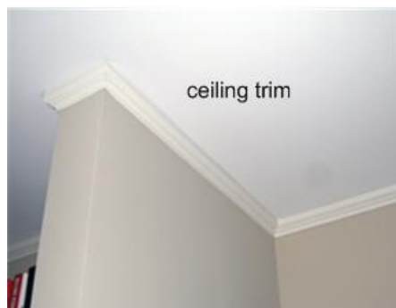
Figure 5. Compound-angle joinery in ceiling and fireplace-mantel moldings
