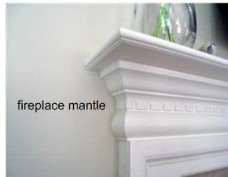
Figure 5. Compound-angle joinery in ceiling and fireplace-mantel moldings
