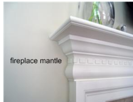
Figure 5. Compound-angle joinery in ceiling and fireplace-mantel moldings
